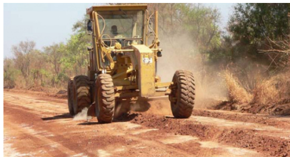
A road construction.
